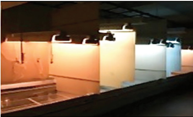
Figure 5.1. This image depicts the various colors of light produced by different fluorescent bulbs. Note the yellow, red, white, and blue colors, all indicating the need to remember that all fluorescent bulbs do not have the same properties. Courtesy of C. R. Raines, The Pennsylvania State University, and M. C. Hunt, Kansas State University.
